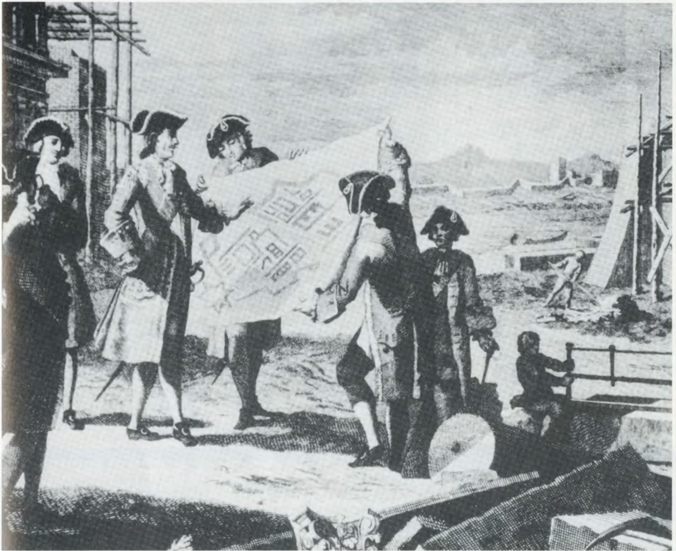
Tsar Peter I supervising the construction of St. Petersburg in 1703; specifically, the Fortress of St. Peter and St. Paul.
