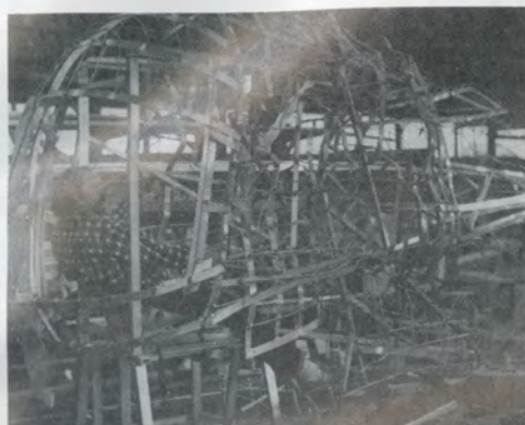
Daniel Nelson of the San Francisco Opera Scenic Construction Shop tries the controls inside the giant skull, while the constructed object is still just a skeleton made of steel.
