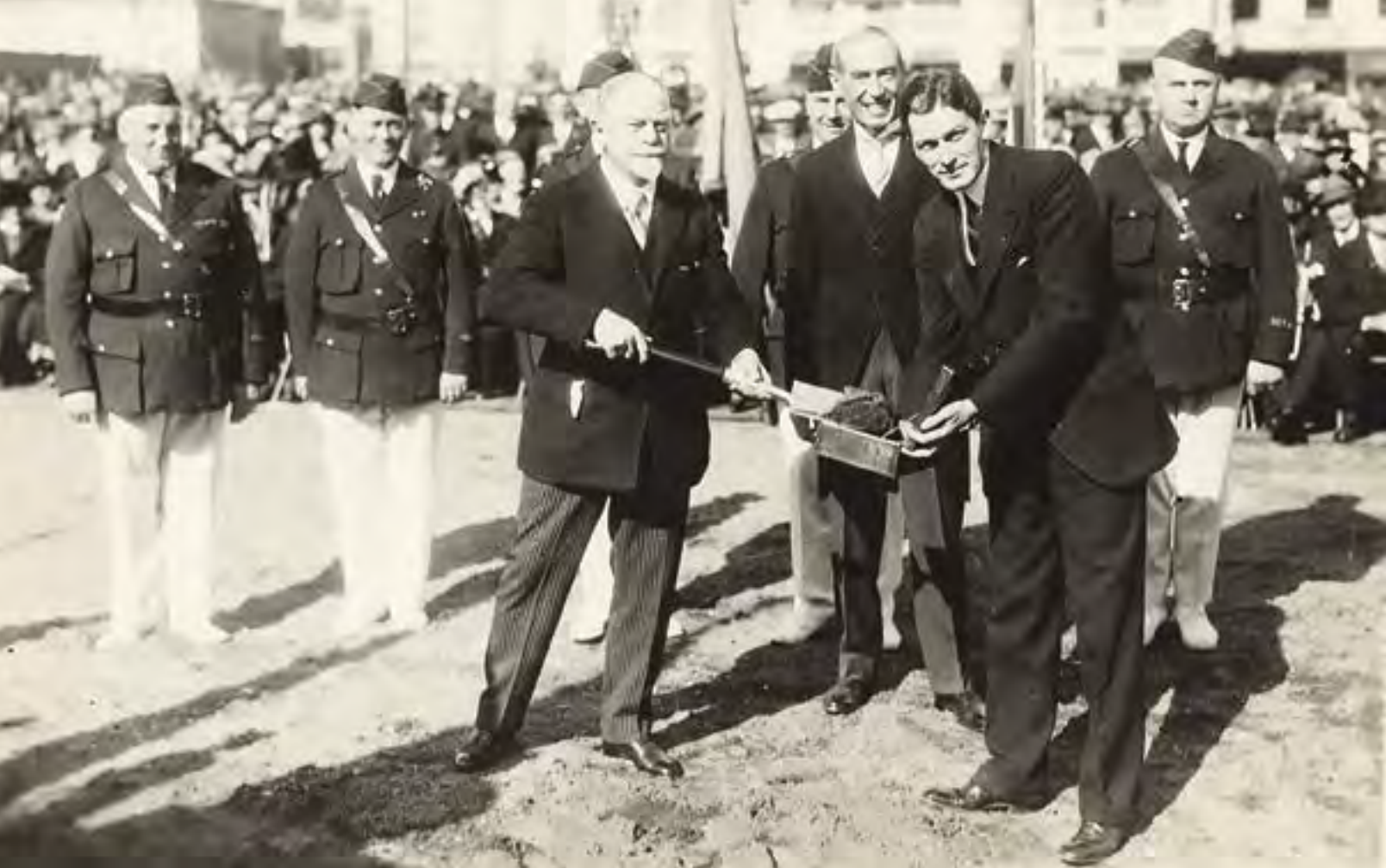
Groundbreaking for San Francisco's new opera house with Charles Kendrick of the War Memorial committee (smiling in the center), November 11, 1926.
