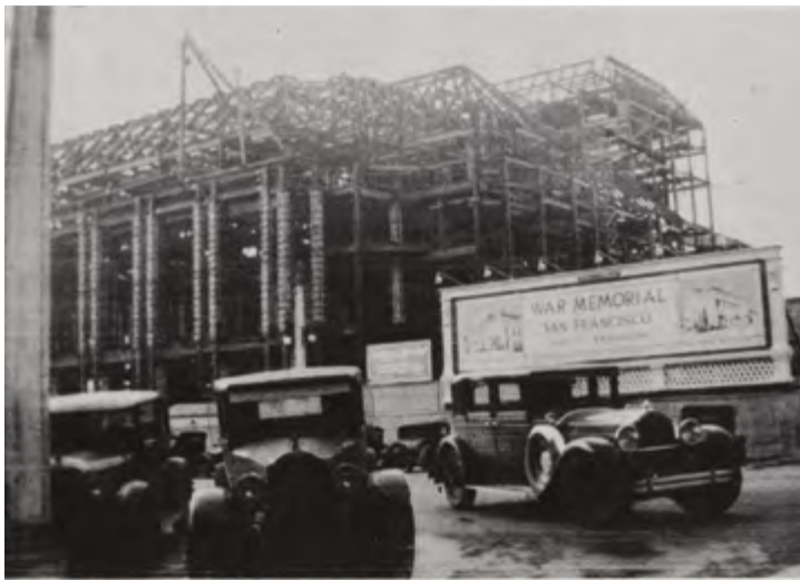
War Memorial Opera House under construction in 1931
