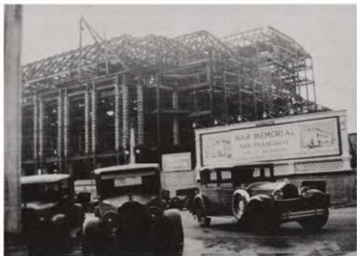
War Memorial Opera House under construction in 1931
