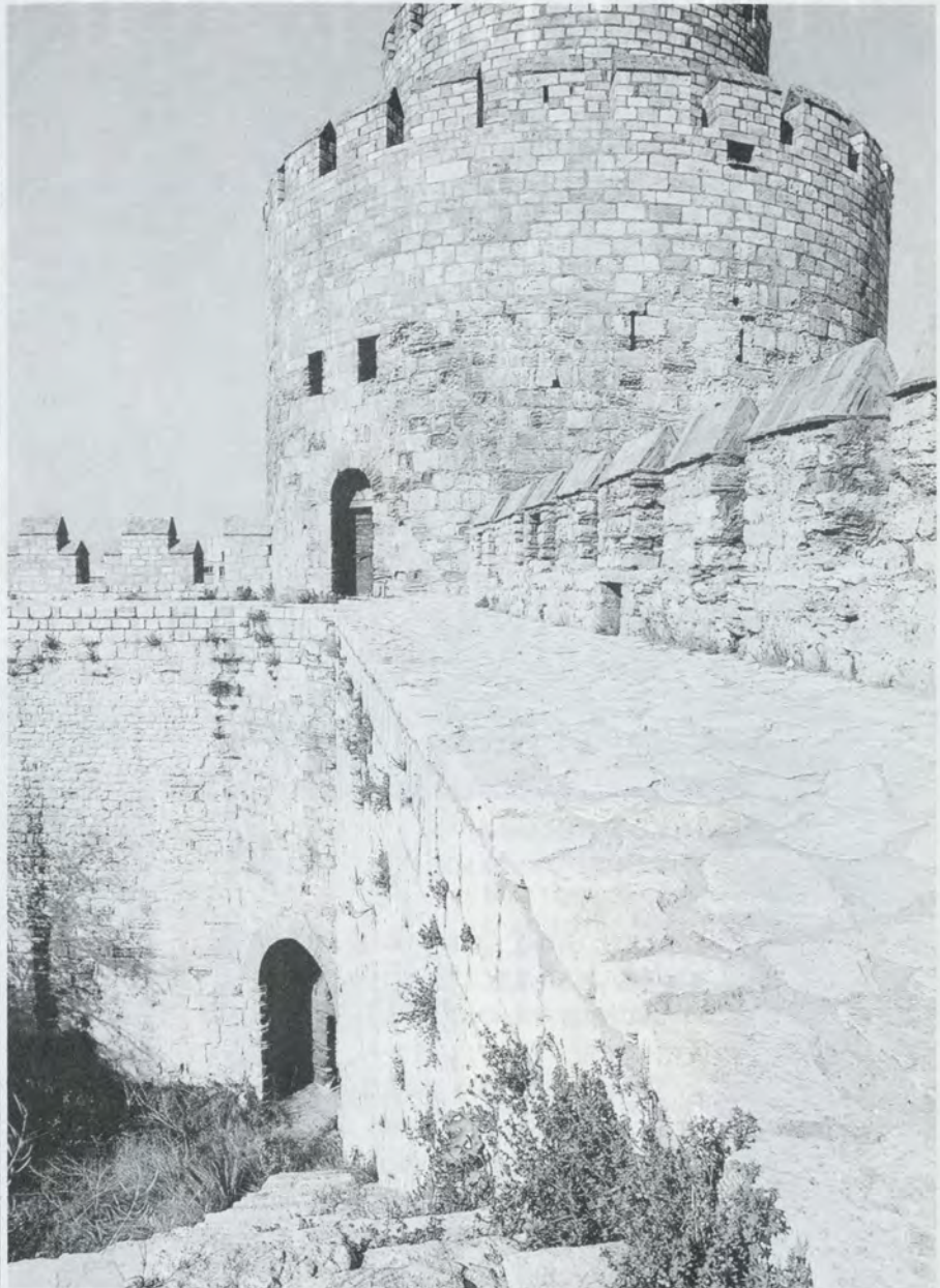
Part of the walls of Constantinople/Istanbul today with a view of the "Seven Towers Castle."
