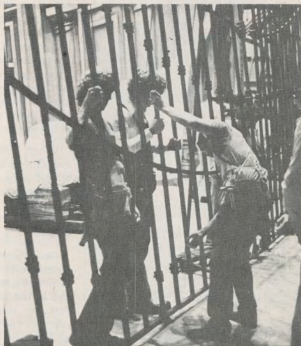
Dan Michalske, Gary Brickley and Nick Bracisco check the iron fence (part of the set seen in the third act) and prepare it for installation on stage.
