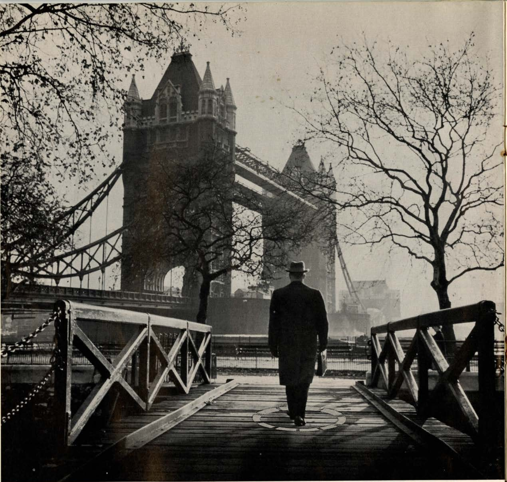
Tower Bridge, London—just two blocks from a Bank of America branch.
